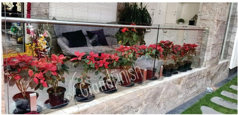
GF 003 Flat Short Baluster System 10x50x200mm with 12mm Toughened Glass
